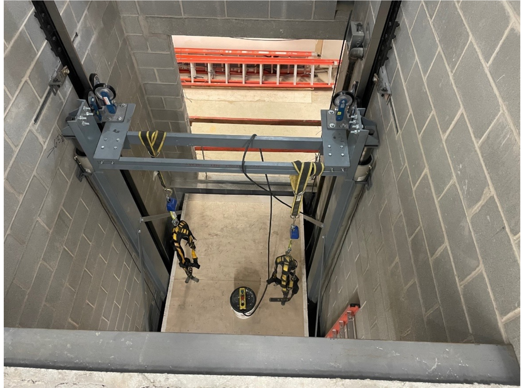
New Stairs and New Elevator
