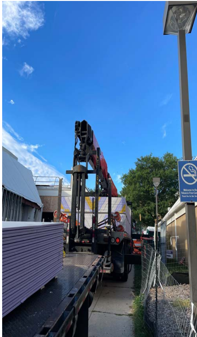
Drywall Delivery Truck
