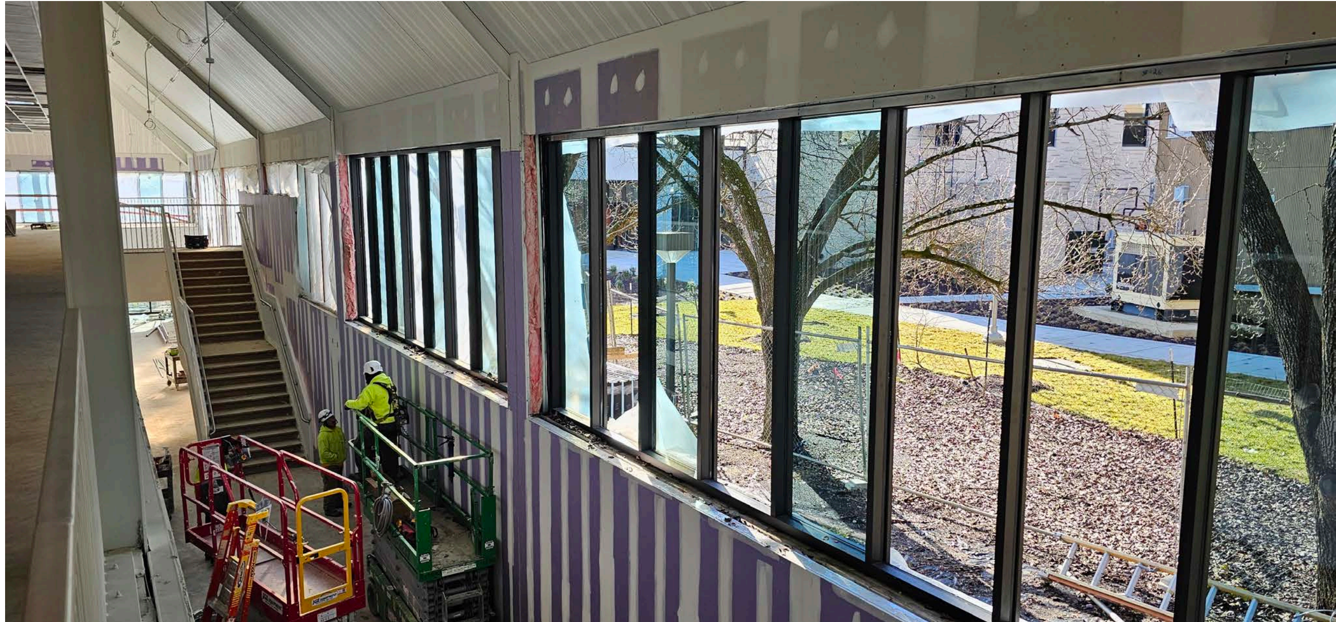
Glass Installation at Windows
