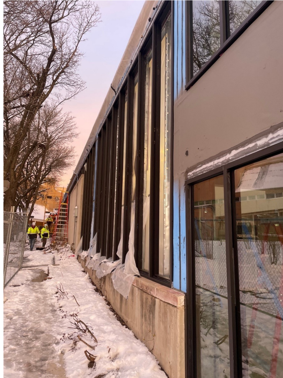
Frames and Glass Installation
