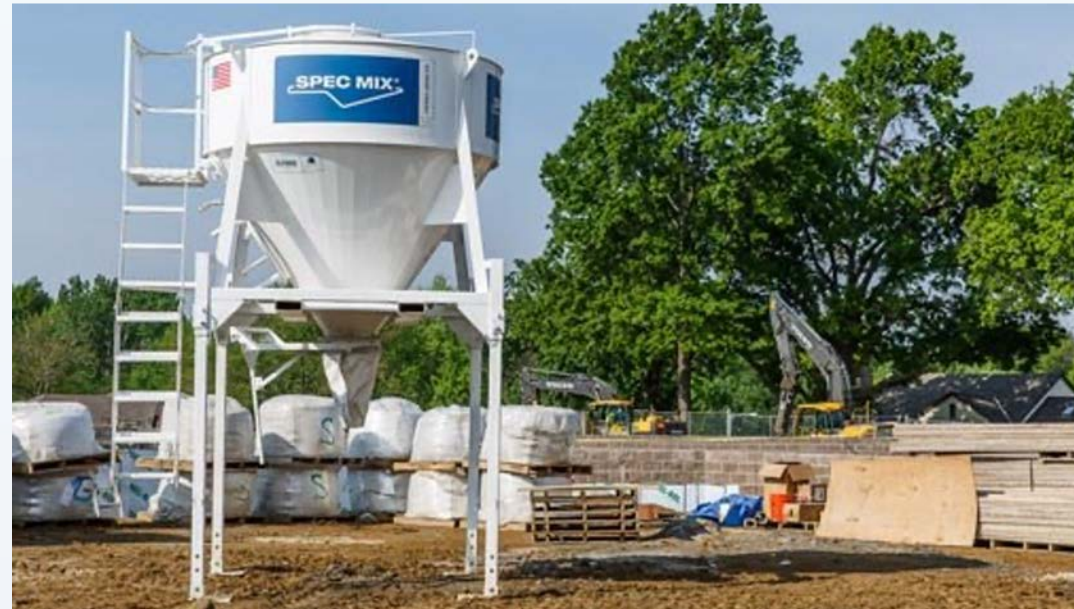
Mortar Storage Silo
