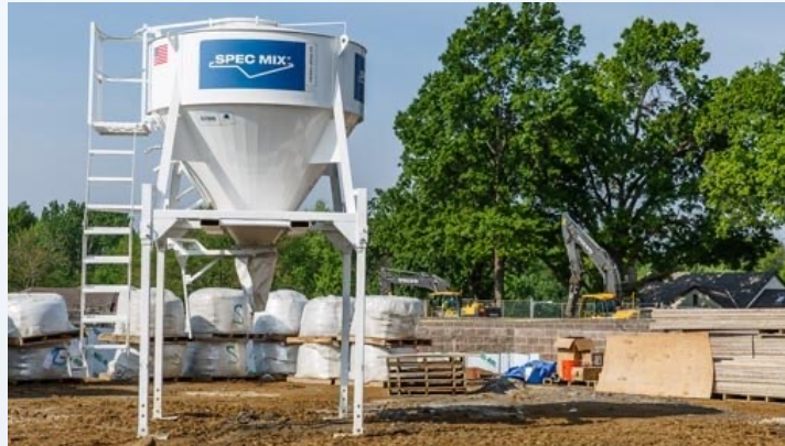
Mortar Storage Silo
