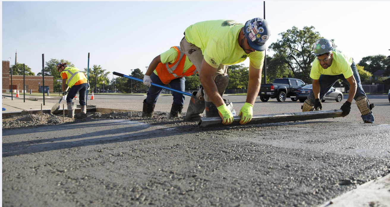
Concrete Finishing Crew
