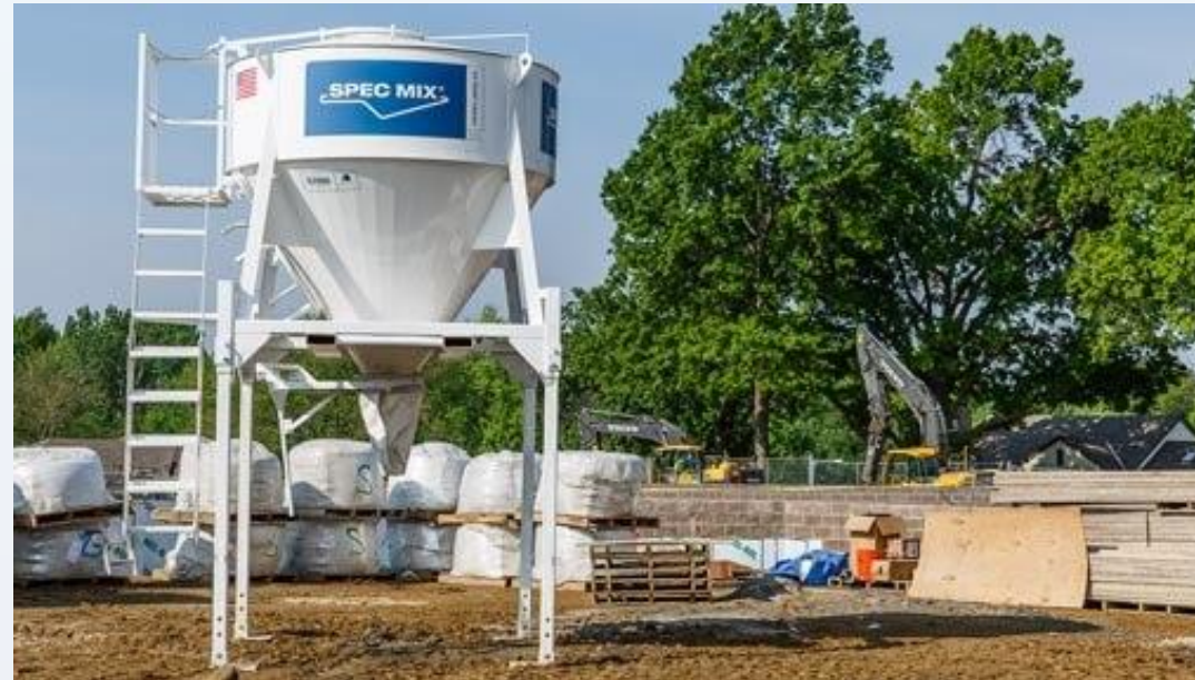
Mortar Storage Silo
