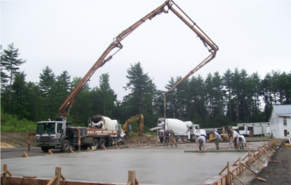
Concrete Pump Truck
