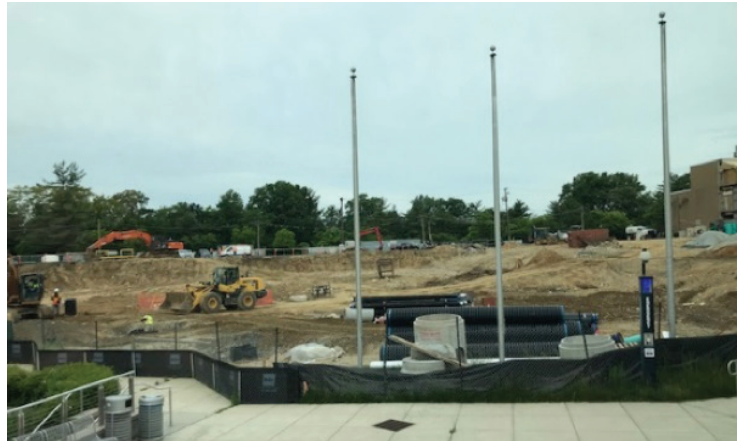
Silt fence with temporary piping to intercept runoff flows.
