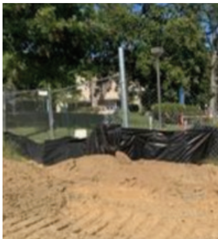
Super silt fence
