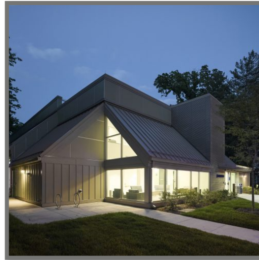
Pavilion 3, Montgomery College Takoma Park/Silver Spring Campus Winner of Montgomery County Planning Department 2017 Buildings and Sites Jury Citations
