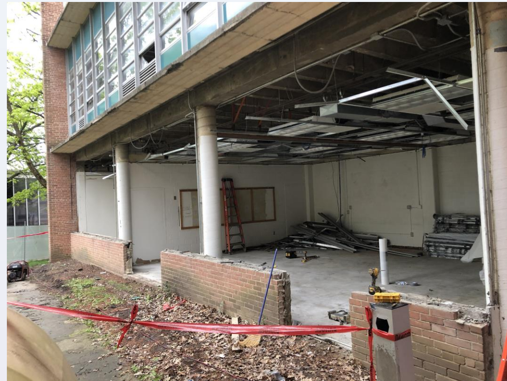
Exterior Window Removal
