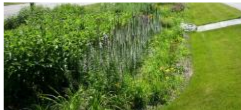
Rain Garden Style Facilities
